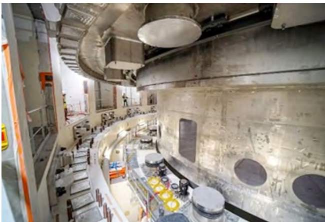
Figure B.3 The Cryostat base section placed with the desired positional accuracy in the tokamak pit
